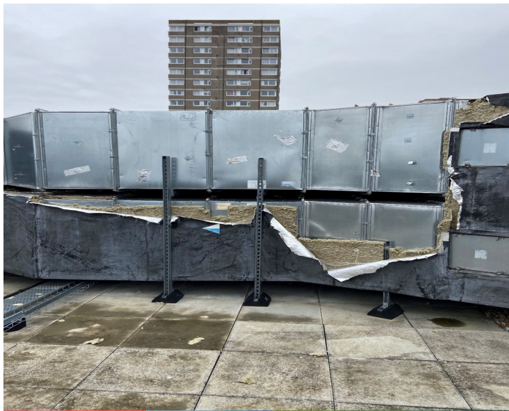
Existing delapidated insulation.
