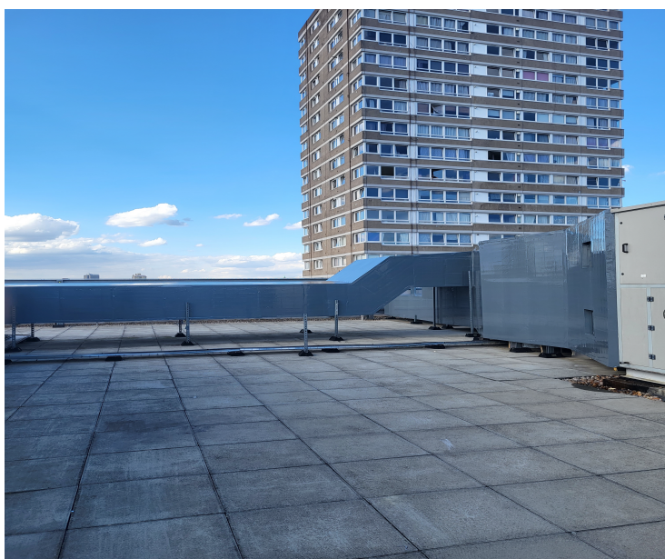
Another view of completed installation of new ductwork installation by Birdsall.
