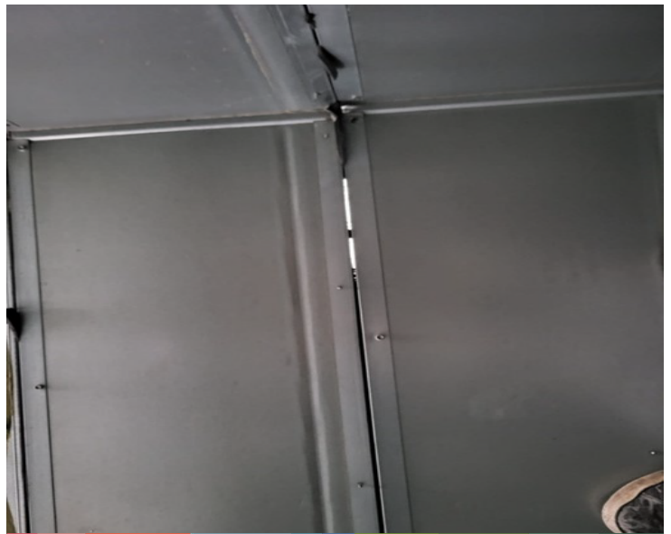
Poorly sealed ductwork joints causing air pressure loss.
